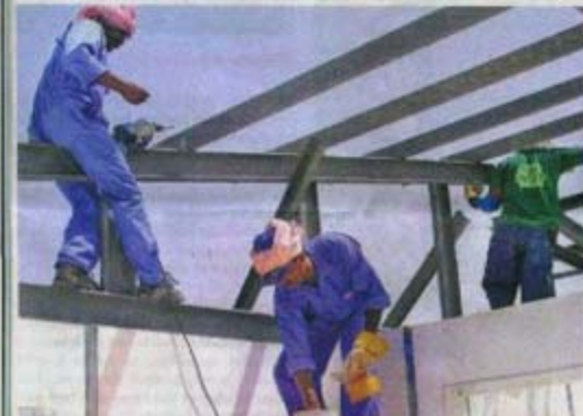
Workers setting up the basic structure of a home near Manila
