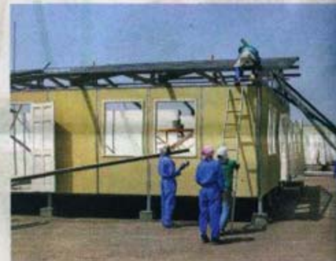
Workers are busy painting the exteriors of a bungalow house
