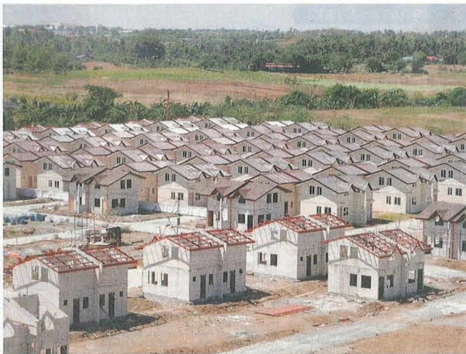
Given the gigantic need for housing in relation to the growing population, brickless technology will be the future of most countries
